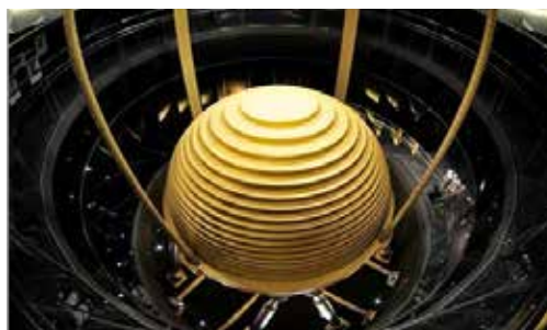
Figure 13 Mechanism of Damping, Taipei 101 Source: www.ctbuh.org/papers
